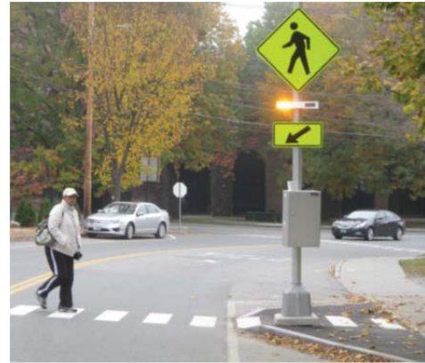
Rapid Flashing Beacon in Hanover, NH
