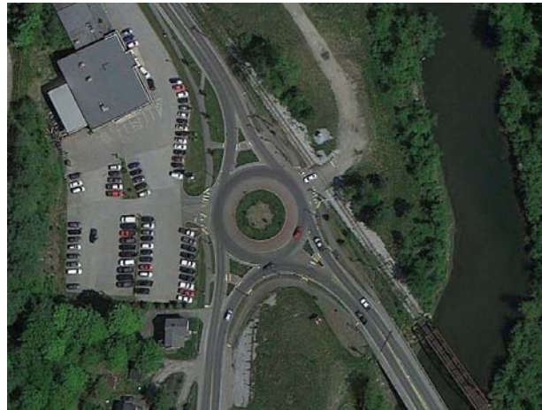
Roundabout in Montpelier at US 2/US 302 intersection
